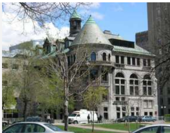
Schulich Library of Science and Engineering ( Macdonald-Stewart Building )
